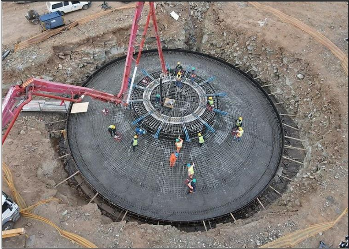
Figure 2.8: Example of Typical Reinforced Concrete Spread Foundations for Wind Turbines (Preliminary Geotechnical and Environmental Geology Report, 2024)
