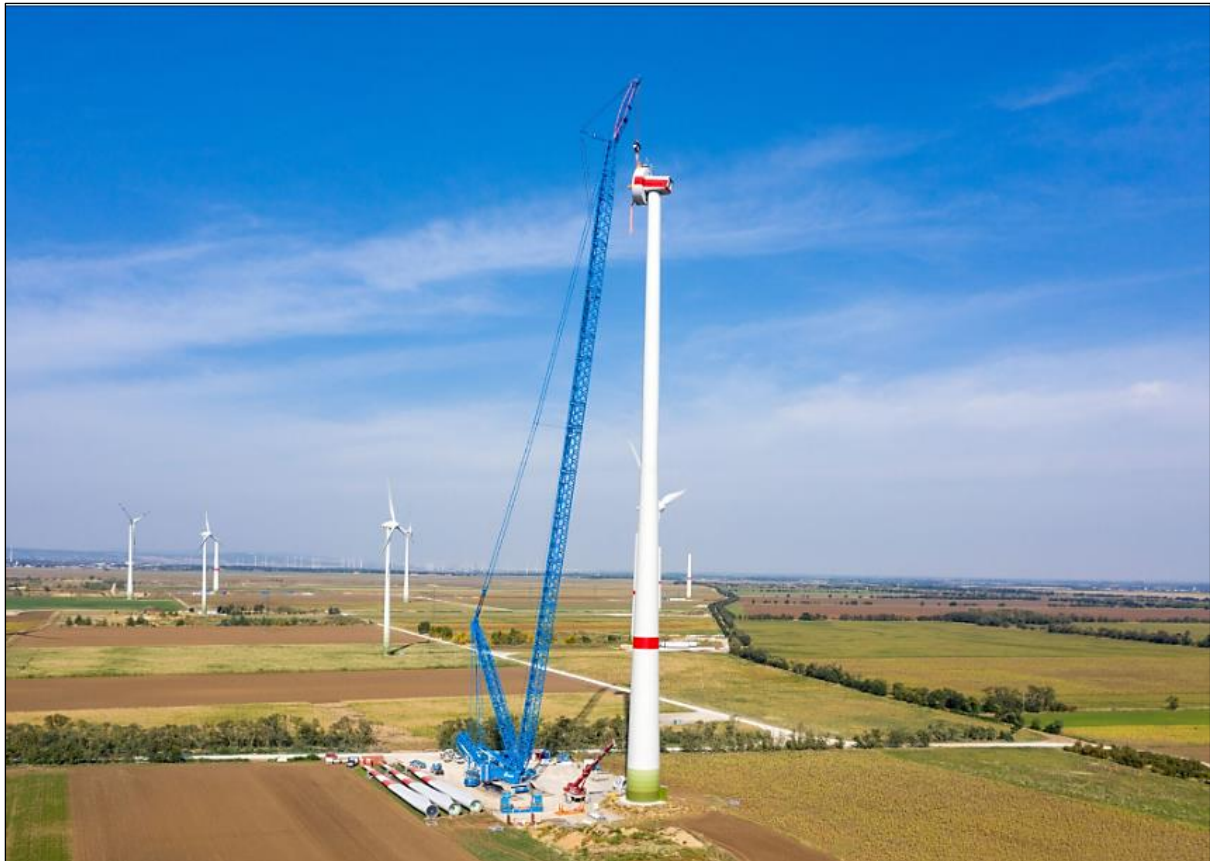
Figure 2.9: Example of Turbine Tower Establishment ( https://www.heavyquipmag.com/2021/11/03/job-story-liebherr-lr-11000-crawler-crane-at-work-to-install-wind-turbines-in-austria/ )
