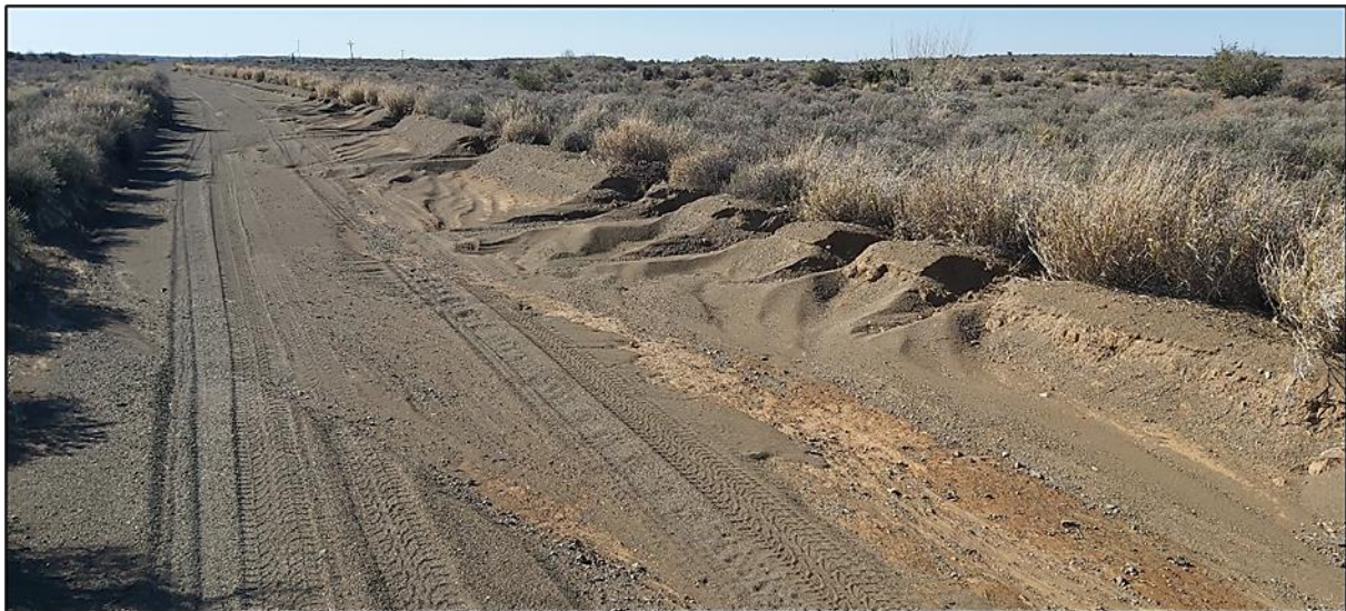
Figure 7.11: Minor Erosion Occurring Where Roads Cross Drainage Lines
